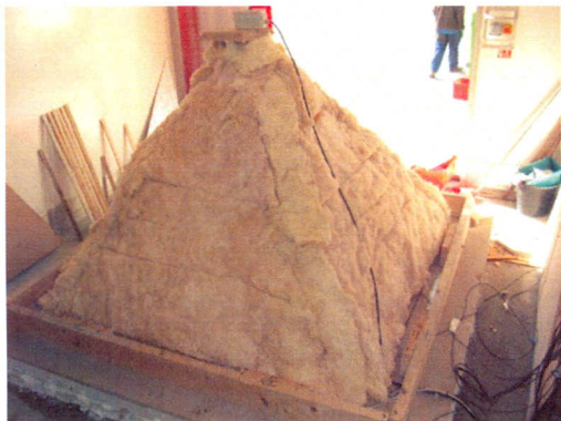
Fig. 3 Glasswool applied over rafters
